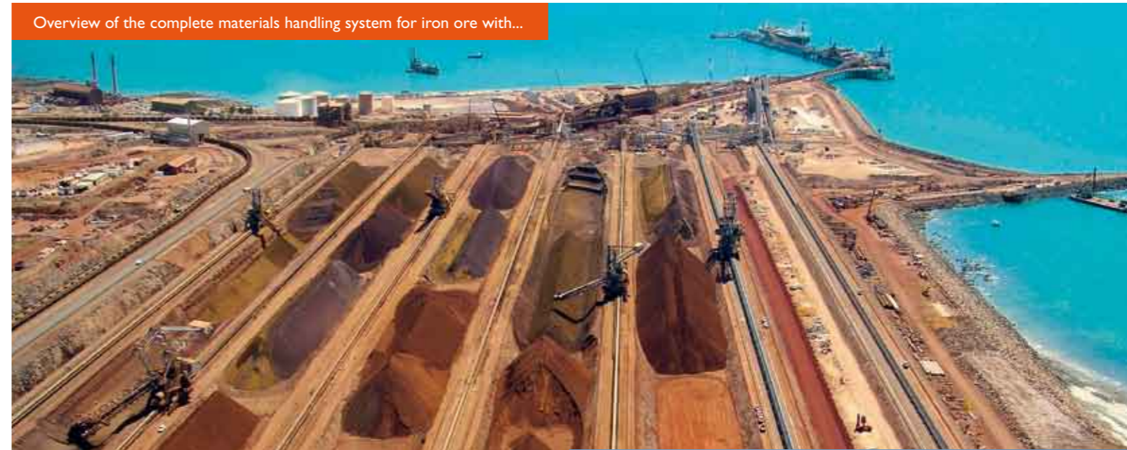
...conveying of the material to the pier...
