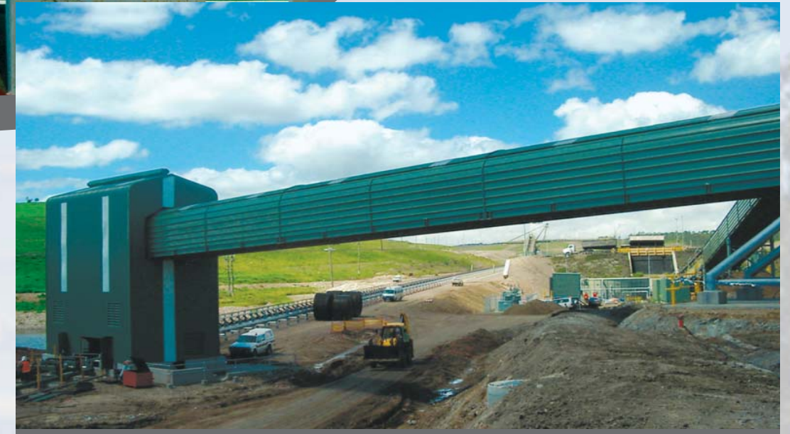
Mt. Arthur North, Overland Conveyor Capacity: 2,500 tph, Length: 1,740 m, Location: NSW, Australia
